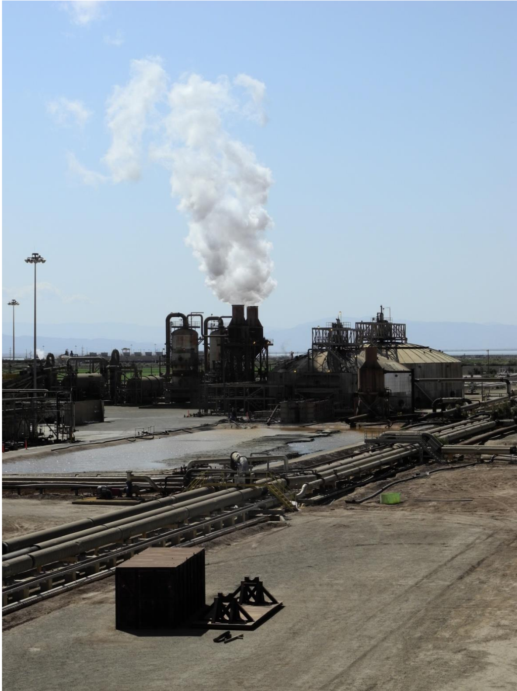
Figure 16: The Geothermal power plant
