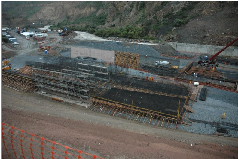
Dam foundations under construction.
